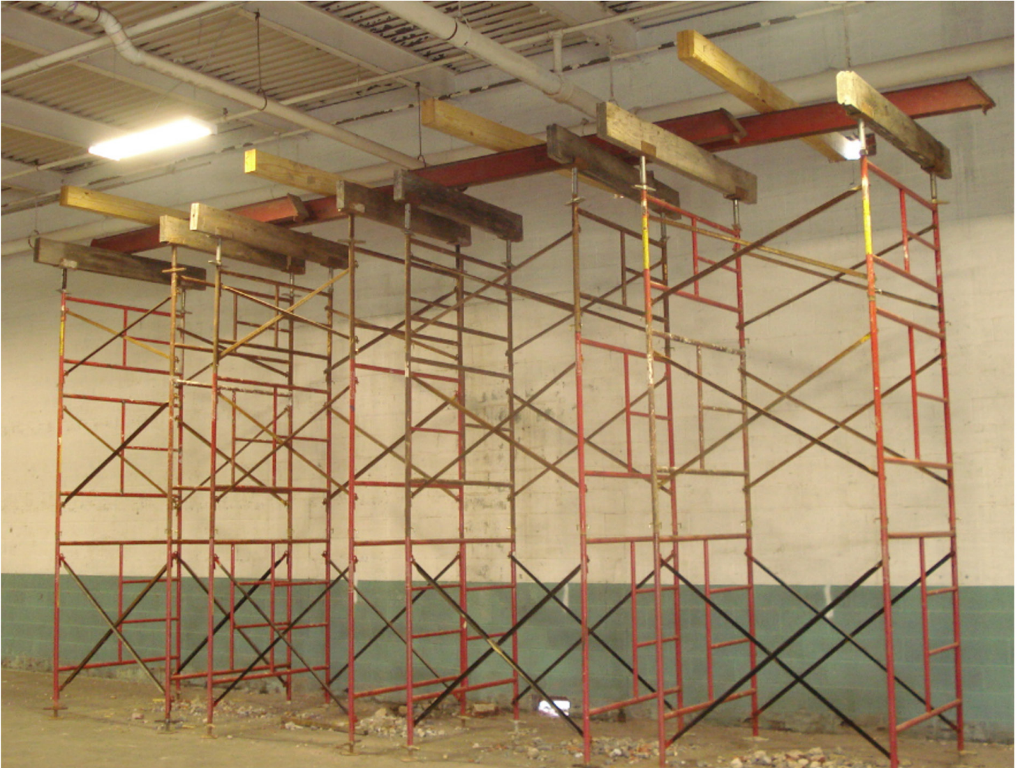
Timber needle beam support of existing CMU wall and existing roof framing members with standard frames.
