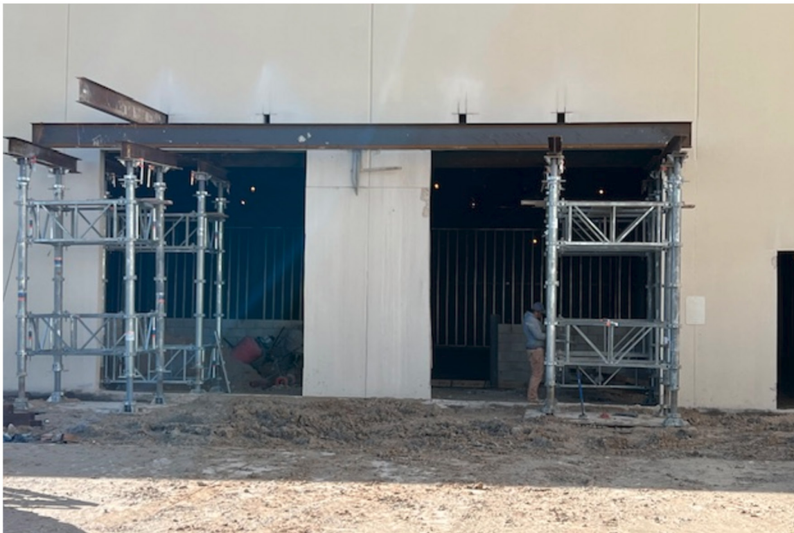
Install progress photo of needle beam support of existing precast concrete panel wall.
