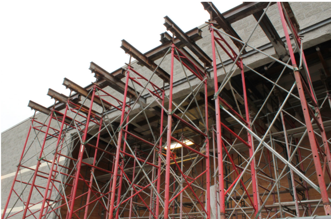
Shoring of CMU wall for new opening. C-channel ledgers to provide additional support of wall were installed along with needle beams and frame shoring.
