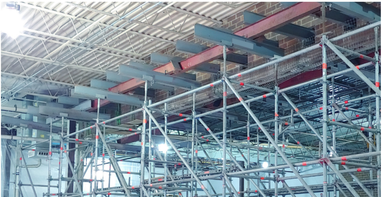
Needle beam support of brick wall and existing roof framing members.
