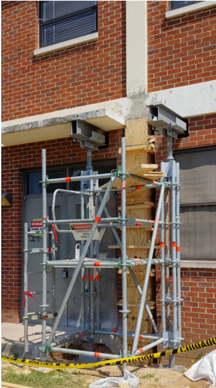
Needle beam support of multi story structure with heavy duty modular shoring tower.
