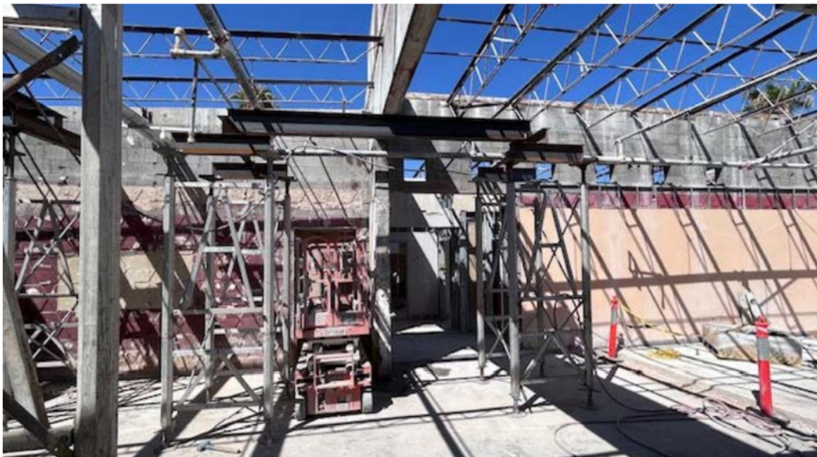
Needle beam with frame shoring towers supporting wall and roof joists.
